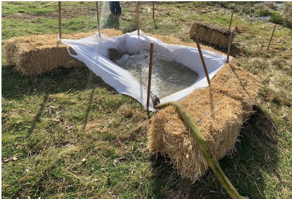
Figure 5: Standard Installation of Geofabric Filter Dam
